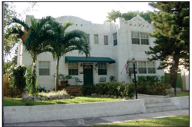
Two-story masonry house in Spring Garden
